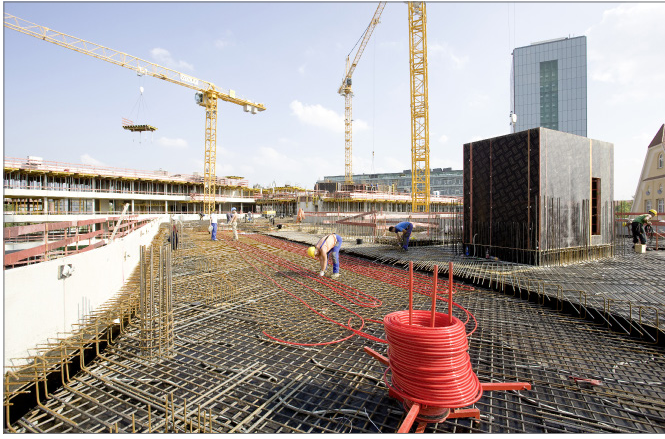
Fig. 2-3 REHAU CCT installed on site
