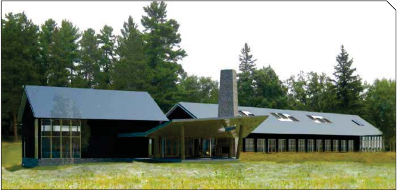
FIGURE 2. The university lab design included a number of energy-saving applications, including a dedicated outdoor air system and photovoltaics. Energy modeling predicted that the building would exceed the proposed energy baseline by 50%.
