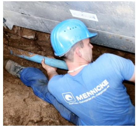
Unconventional method: A claw was attached to the pipe to grip it securely due to the rapidly compacting sand. This posed no problem for the notch and point-load resistant REHAU PEXa pipe.
