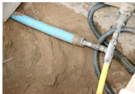
Successfully installed REHAU PEXa potable water service pipe
