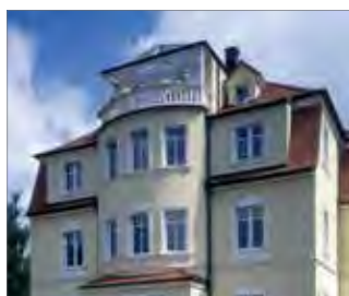
Klasa 2: stary budynek po remoncie Q = 85 - 115 \text{ kWh}/(\text{m}^2 \cdot \text{a})
